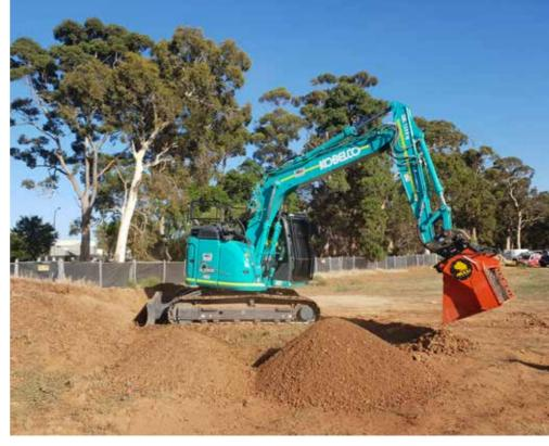
'vibrating screening' method. Vibrating screening is a time-consuming two-stage process with high fuel consumption, particularly when using the smaller screen.
